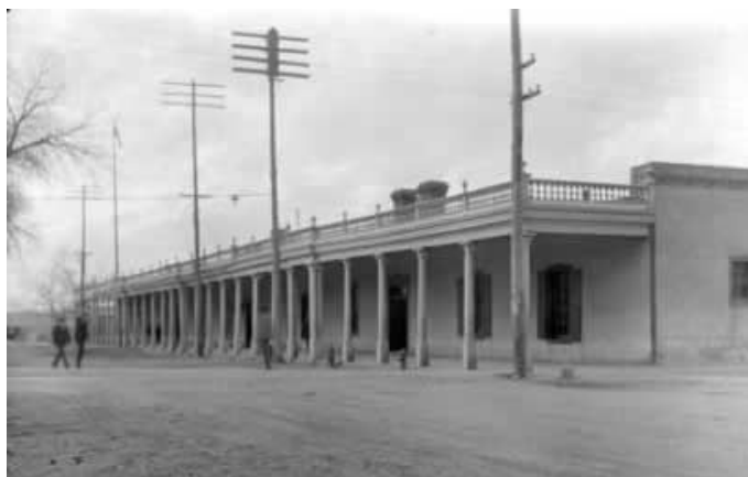
One of the oldest buildings in Santa Fe, the Palace of the Governors, with its added portal.
